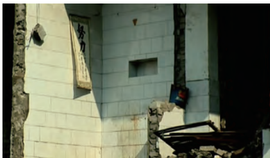
Figure 13 Calligraphy and Painting “Efforts” in the Ruins of the Demolition
